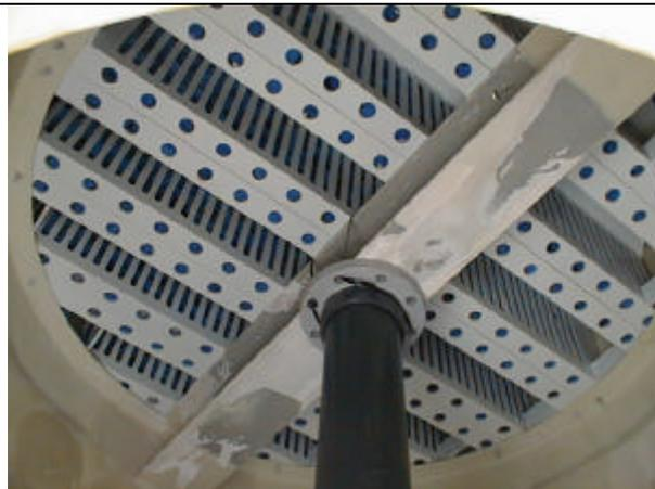
Reinforcement of the packing support in biotrickling filter 10. Subsequent conversions did not include such a reinforcement.
