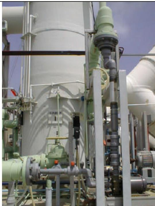
Biotrickling filter I at Plant 2 which treats very high  $H_2S$  concentrations (roughing biotrickling filter).
