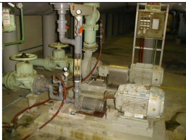
Recycle pump for biotrickling filter G. The former pump is on the right, smaller pump installed on the left.
