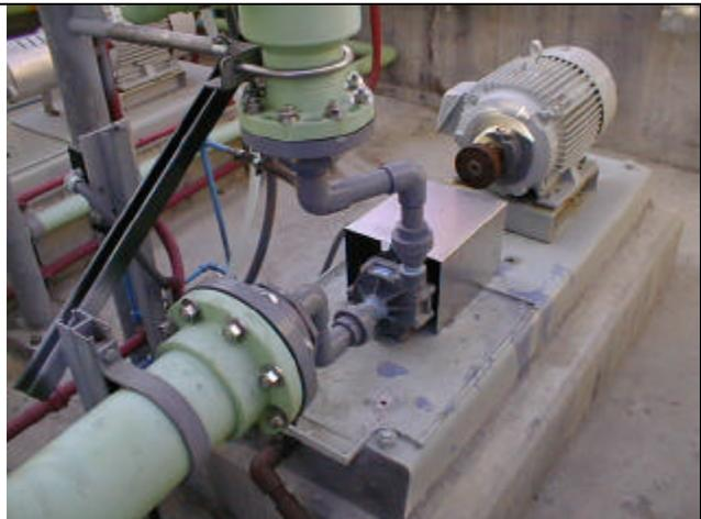
Because trickling rate is much lower in biotrickling filters, a smaller recycle pump (shown under protective cover) was installed on biotrickling filter 10. The larger pump is shown in the back.
