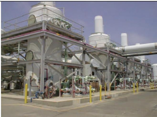
North Complex at Plant 2. The second scrubber from the left is biotrickling filter Q which treats part of the air from biotrickling filter I.
